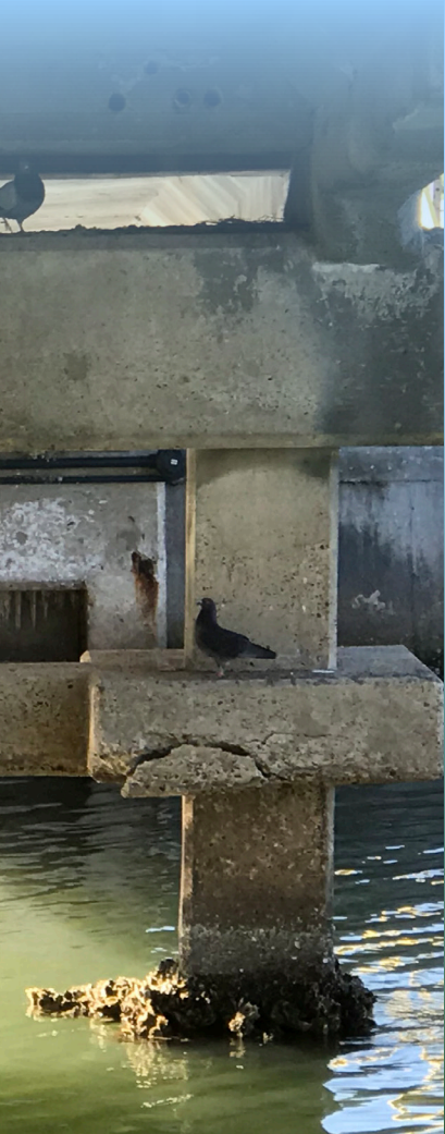
Figure 5: Visible Concrete Deterioration
