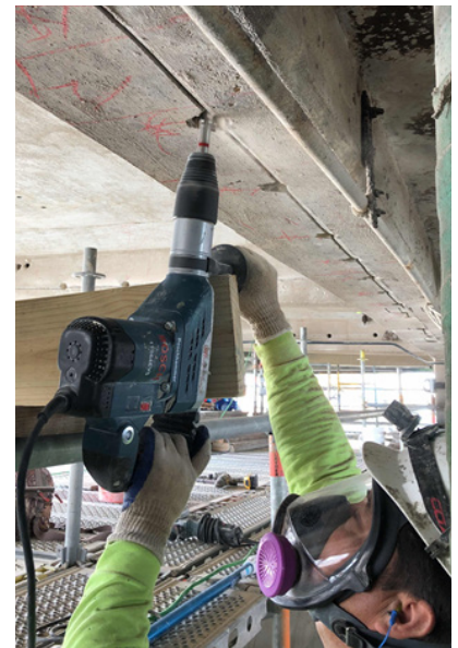
Figure 15: Drilling Overhead on Upper-Level Beams
