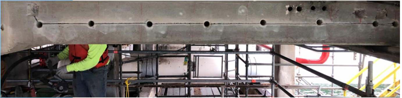
Figure 8: Drilling Anode Holes
