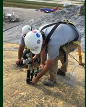
*Impact echo/pulse velocity testing of a hangar at the Kansas City Airport*
