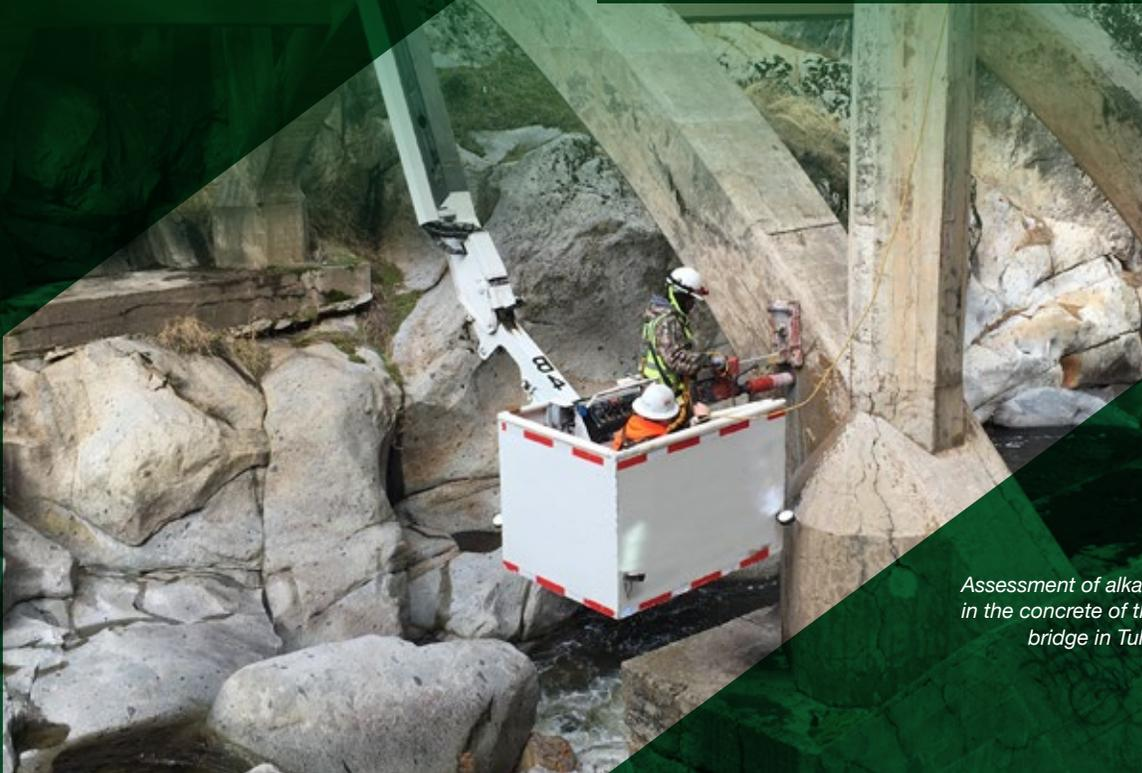
*Assessment of alkali silica reaction in the concrete of the Mineral King bridge in Tulare County, CA*
