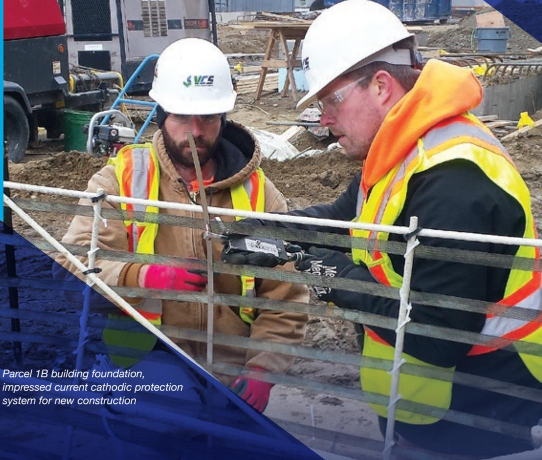
Parcel 1B building foundation, impressed current cathodic protection system for new construction
